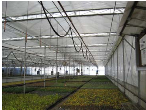
Thermal screens partially open to allow solar gain on a cool, cloudy day in December
