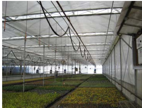
Thermal screens partially open to allow solar gain on a cool, cloudy day in December
